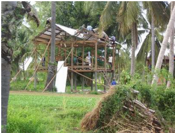
Communal house building. Krosang
